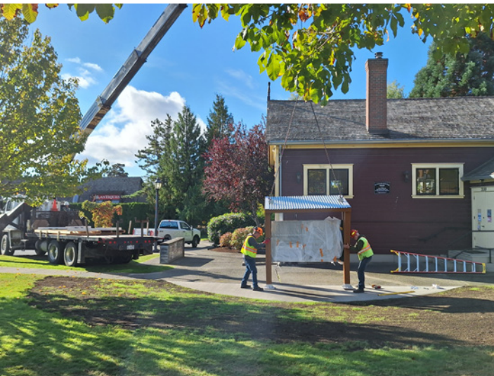
Installation of the information kiosk in HEL,HILEĆ
