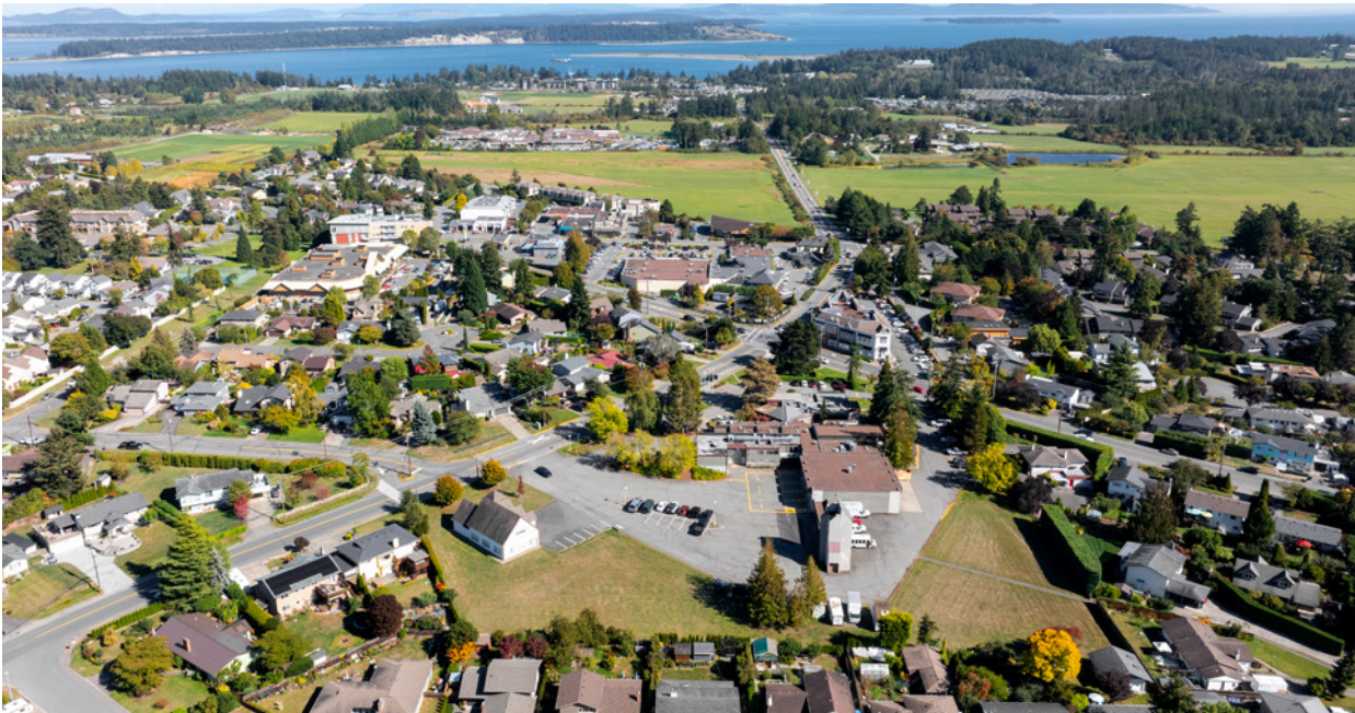
Aerial photo of 1903 Mt Newton Cross Road
