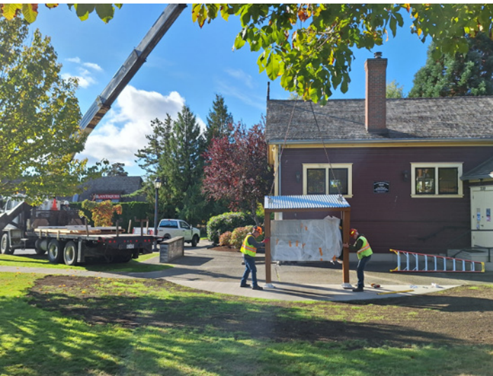
Installation of the information kiosk in HEL,HILEĆ
