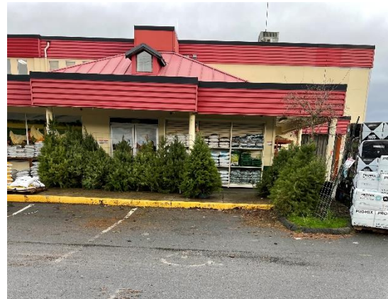
Example of an accessible space with faded paint
